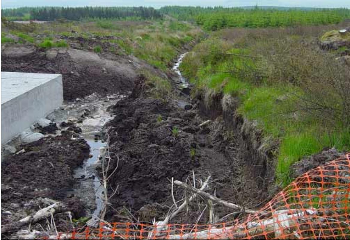
**Plate 9.1: The excavation at T17 lies on the line of an already-existing double ditch and so is well drained. Nonetheless, it was the site of the first substantial bog slide.**
