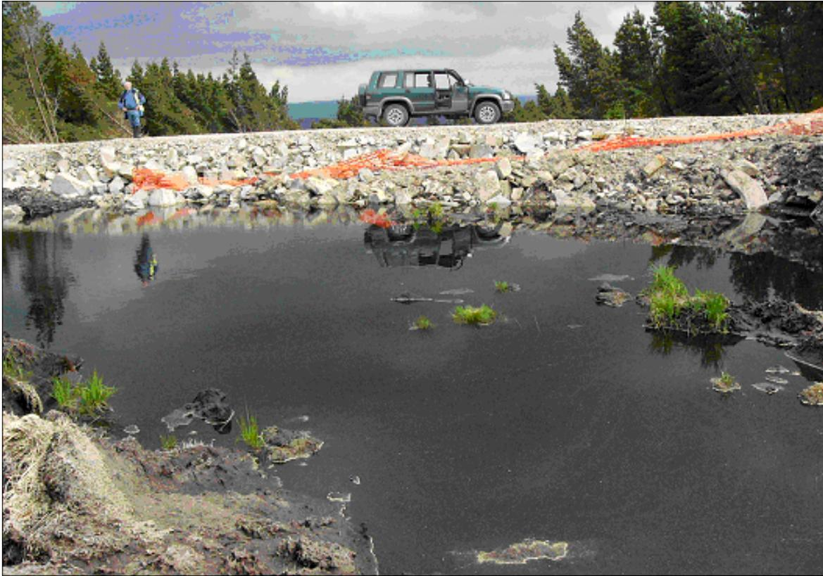
**Plate 8.11: A damaged floating road just by T68. By June 2004, when this photograph was taken, it had been top-loaded with some decimetres of rock and aggregate, presumably rendering it rather less permeable to water than previously. A considerable depth of water had accumulated upslope, as the picture shows.**
