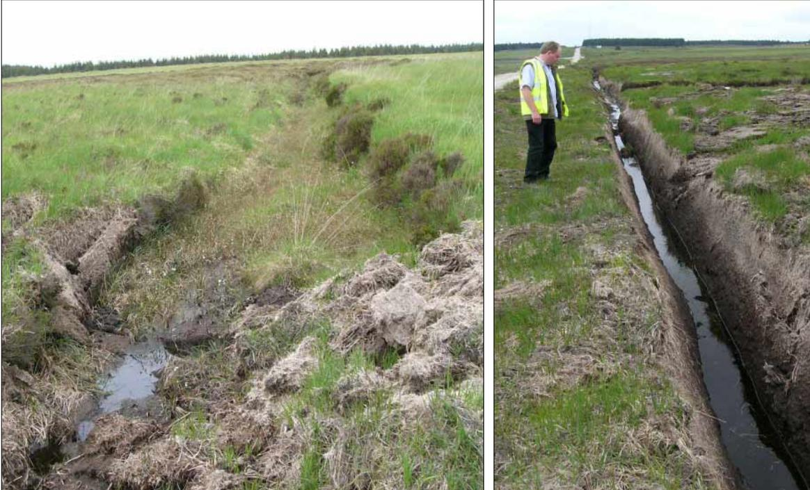
**Plate 3.6:** Turbarry fields on the summit of the site showing (above) an old peat bank and (right) the downslope catchwater drainage system, re-excavated after peat slide in 2003).
