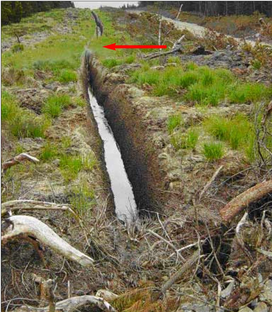
**Plate 10.2:** A ditch that runs ENE from T53 alongside a floating road across the northern slope of the mountain has obviously bowed and slumped downslope where it crosses deep peat. (It is assumed it originally ran straight.)
