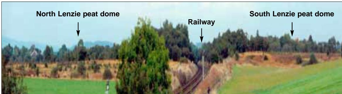
**Plate 5.2:** Railway line ‘floated’ across Lenzie Moss during the 19th Century. The track has now sunk by about three metres and the bog is clearly divided into two sections. Note also the lines of taller trees flanking the track, reflecting the associated drainage.
