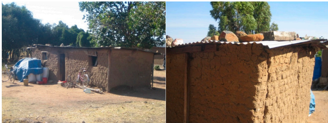
Figure 2. A low-income house with clay walls and an iron sheet roof.
