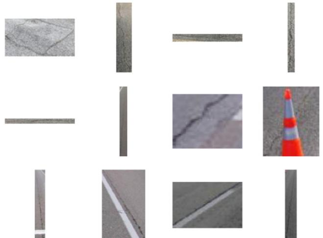
Fig. 4. Collage of Images in the Longitudinal Crack Category
