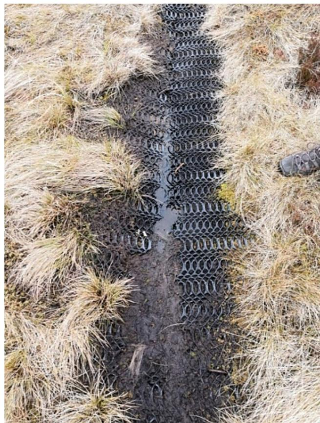
FIGURE 5 Area of failed track in a rutted section.
